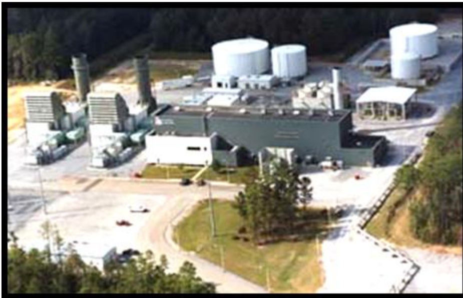
Figure ES-2 110 MW – 26 hr 1 st generation CAES system at Alabama Electric Cooperative
